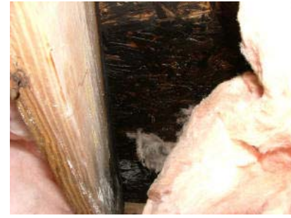
Harbor Place, James Island, SC - The subfloor under these hardwood floors was saturated causing the floors above to buckle.
