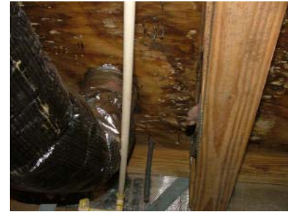
Millbrook Court, Longpoint, Mt. Pleasant, SC - Widespread cupping of the hardwood floor in this Mt. Pleasant home was caused by elevated crawl space moisture.
