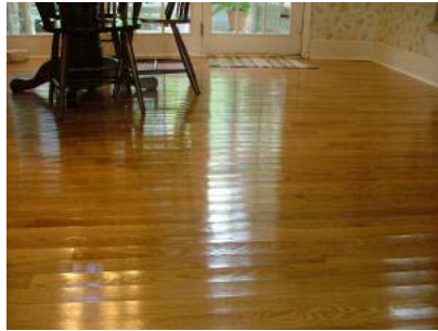
Millbrook Court, Longpoint, Mt. Pleasant, SC - Widespread cupping of the hardwood floor in this Mt. Pleasant home was caused by elevated crawl space moisture.
