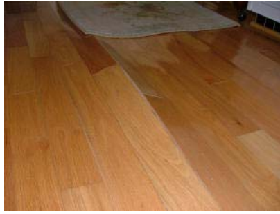
Harbor Place, James Island, SC - The subfloor under these hardwood floors was saturated causing the floors above to buckle.
