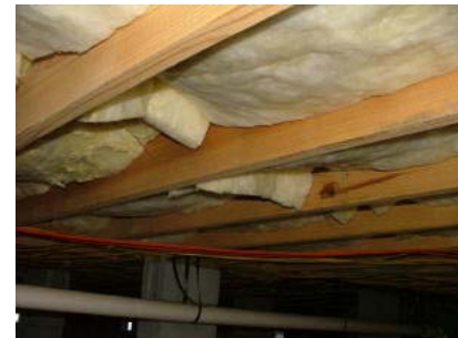
Clearspring Drive, Ocean Neighbors, James Island, SC - Although the crawl space of this James Island home appeared dry, the elevated relative humidity (as compared to that on the inside) was enough to cause these floors to cup.
