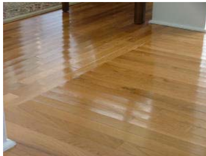
Clearspring Drive, Ocean Neighbors, James Island, SC - Although the crawl space of this James Island home appeared dry, the elevated relative humidity (as compared to that on the inside) was enough to cause these floors to cup.
