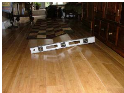
Monico Drive, Townhomes of Beaumont, Mt. Pleasant, SC - The moisture content of the slab below these floors was high enough to cause these hardwoods to buckle. The
